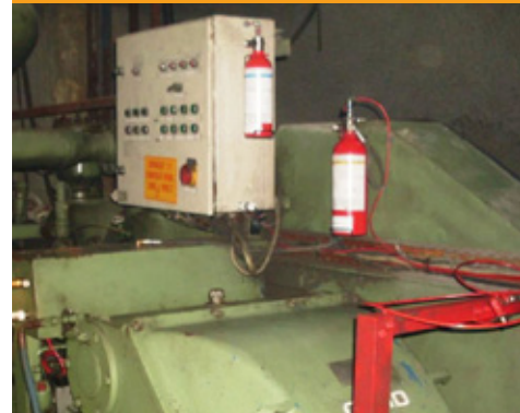
A Firetrace system can prevent a small fire from becoming a major event.
